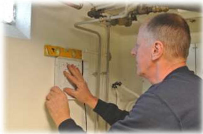
Roy Lindström, fiberinstallation hos kund.
